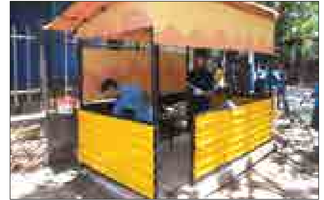
Renovation of Bus Halt
